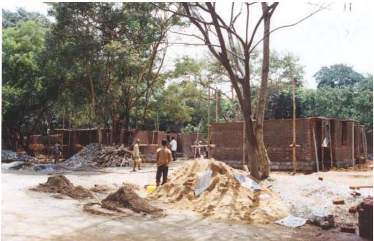
Quarters under construction
